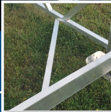
CORNER BRACES FOR STABILITY
